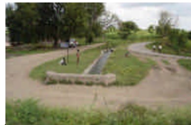
Mula Minor 7 under the control of the society to distribute the allocated water
