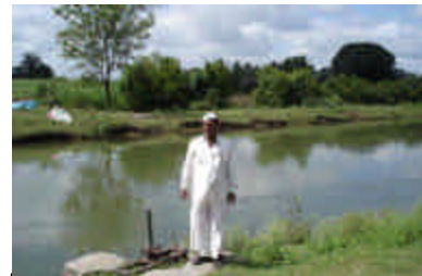
Main sluice gate to release allocated quota of Mula river water
